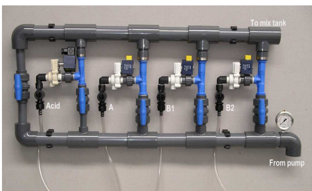
Typical injection manifold
